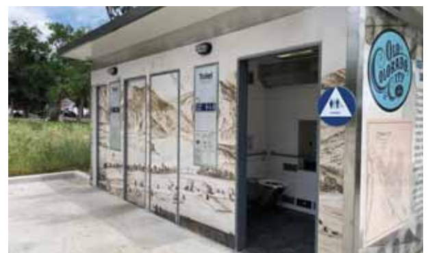
Public Restrooms with Visitor Information, Bancroft Park, Colorado
