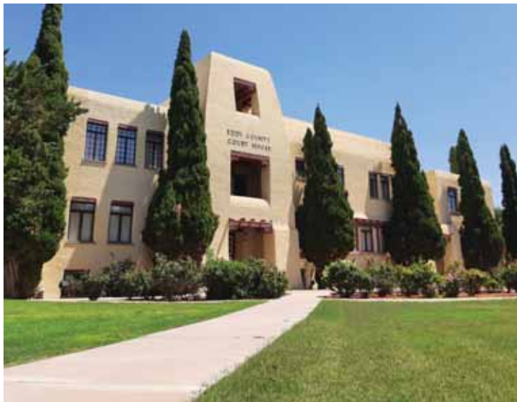
Eddy County Courthouse Lawn
