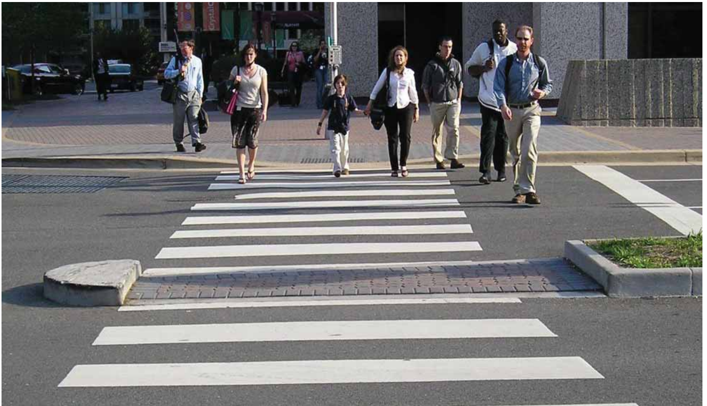
Continental" crosswalk pattern with an extended median - National Association of City Transportation Officials
